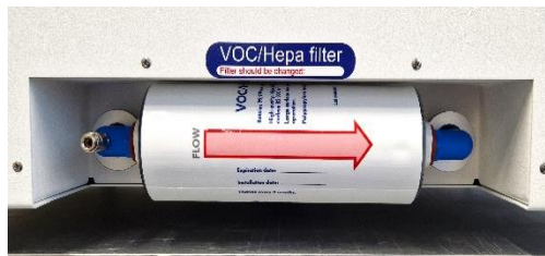
Figure 12.3 Correctly installed VOC/HEPA filter
